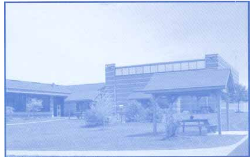
Dual Jurisdiction Facility - Montgomery City
